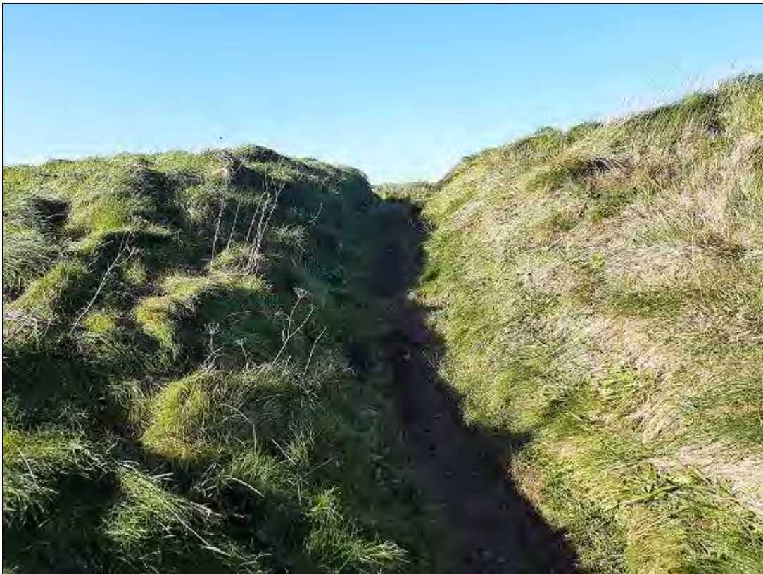
Plate 2. Detail of deep groove caused by pedestrian footfall on S face of motte, from S.
